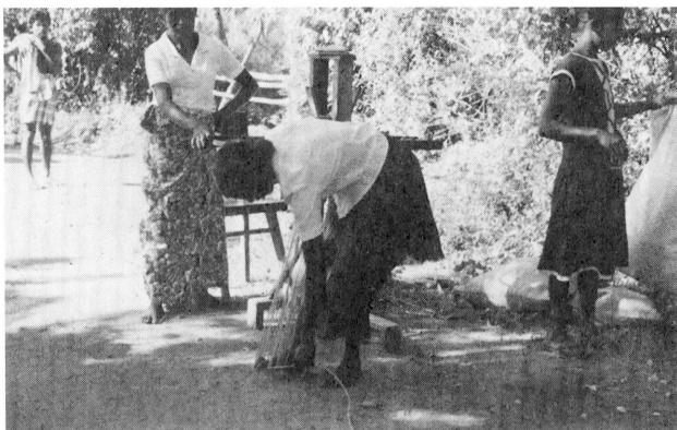
Coir yarn making from coconut husks
